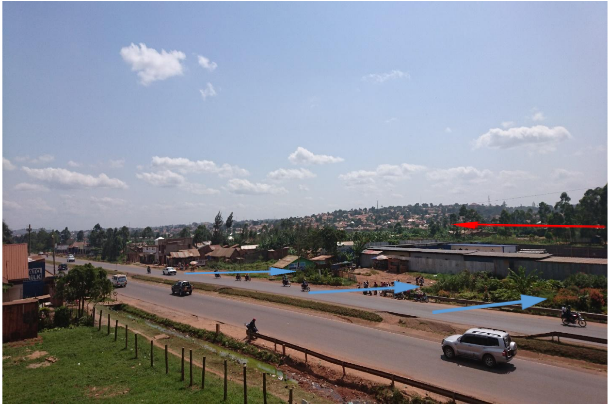
Figure 6 the blue arrows illustrate how water flows into the Kawaala community when it rains because there is an improper drainage system along the Northern By-Pass. The red arrow shows the direction of the diversion.
