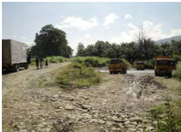
Picture 26: Company Trucks Repairing Sections of Kokoda National Highway
