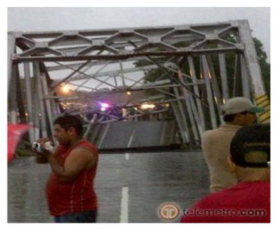
Figure 6 – Bridge collapsed on the Pan-American Highway due to floods (Foto Telemetro.com)
