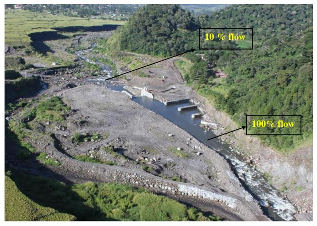
Figure 1: Example of an existing dam shown by the Requesters to the Panel and demonstrating the difference between full flow up-stream and 10 percent flow down-stream from a dam (Source: Damaris Sanchez, Requester).
