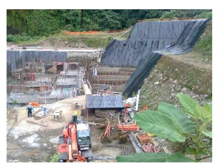
Figure 5 – Erosion control during construction of PML
