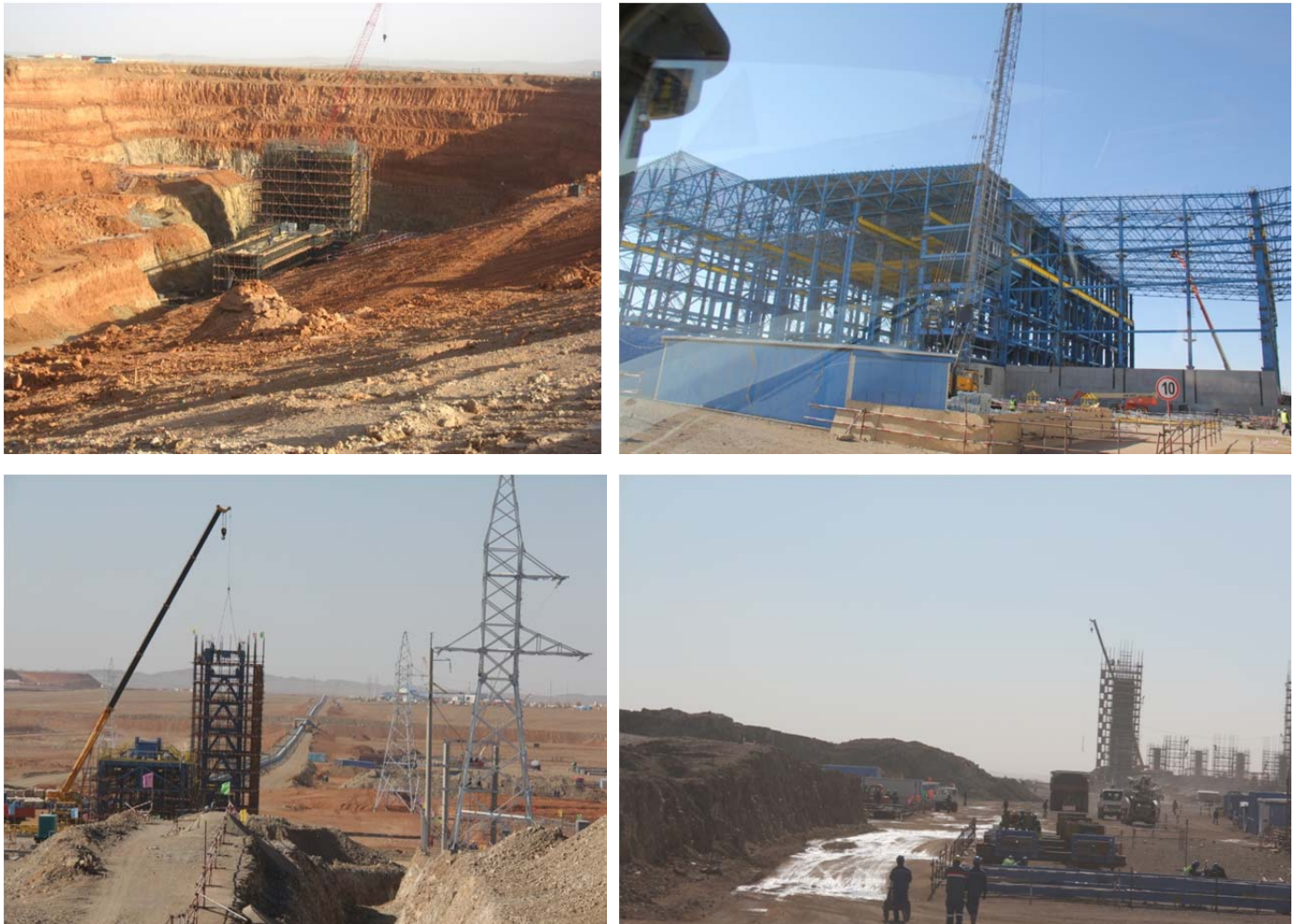
Figure 8. Construction activities at OT site, May 2011.
