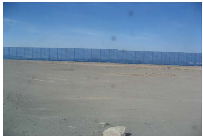
Figure 4. Fencing by one company along one side of its coal yard.
