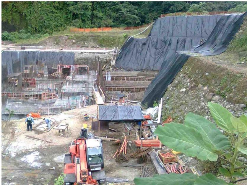
**Figure 5 – Erosion control during construction of PML**
