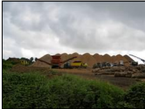
BR's woodchip stockpiles in the Port of Buchanan. Smoke can be seen rising from the tops of the piles, indicating that the woodchips are decomposing.
